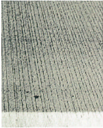
25 mm Uniform Skew 1:6 RHF ETD = 0.334, d = 1.2, w = 4.1
