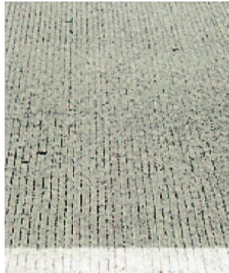
R3 Hw. 26, 25 mm Random Transverse ETD = 0.952, d = 2.6, w = 6.5
