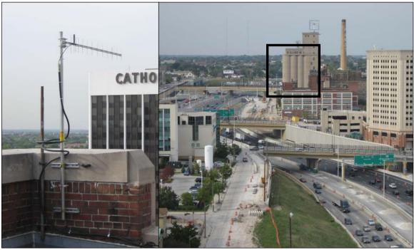
Figure 3-20 - Left: The wireless antenna mounted on the corner of Carpenter Tower Hall at Marquette. Right: View from the antenna location at Carpenter Tower. The test section is located just behind the grain elevators in the highlighted area.
