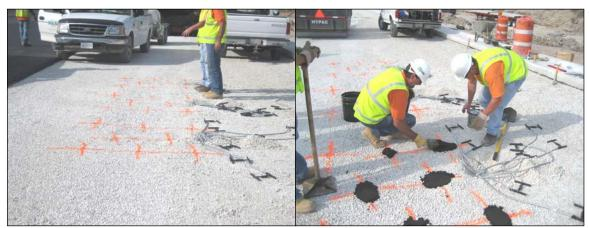
Figure 3-15 - Left: Marking the proposed locations of the gauges. Right: Placing sand/binder pad and fitting gauges.
