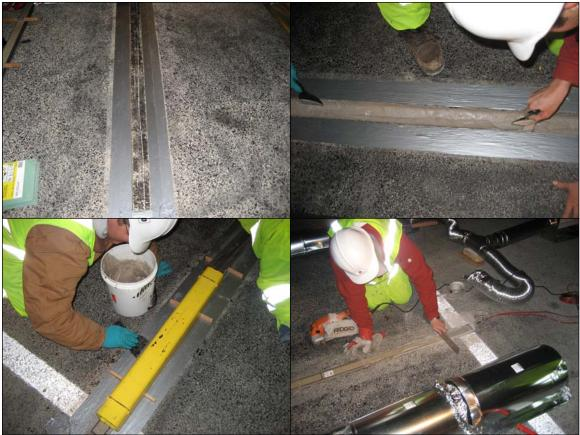
Figure 3-26 - Upper left: Channel for the WIM sensor ready for installation. Upper right: Grout for the sensor being distributed into the channel. Lower left: Sensor in place with pieces of steel placed across the leveling beams to keep sensor from floating out of the grout. Touch up work to the grout was done before its initial set. Lower right: The sensors were ground flush with the surrounding pavement and checked using an 18-inch long straight edge.
