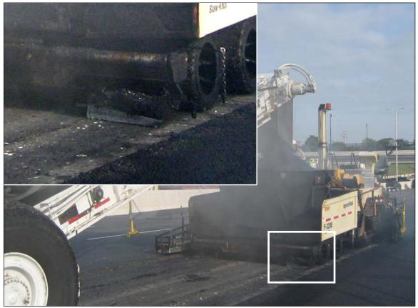
Figure 3-22 – The scraper in the wheel paths of the pavers should be lifted off the pavement surface to avoid destroying sensors and their wiring. The inset picture is a close-up of the scraper which is in the down position, resting on the pavement surface.
