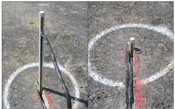
Figure 3-21 - The photograph on the left shows almost the entire length of the temperature probe. The photograph on the right shows the temperature probe fully inserted to its final position. Note that the sensor lead is fitted into its channel, but has not been sealed yet.
