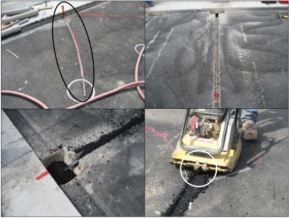
Figure 3-36 - Installation of the WIM, wheel wander, and temperature sensor conduits. Top left: Grooves were cut with a saw for the sensor leads for the pavement temperature gradient probes. Top right and bottom left: Groove cut with conduit in place for a WIM sensor. Bottom right: Asphalt being re-compacted into groove cut for the wheel-wander sensors. The plate tamper had a bolt-on bar (circled) mounted on the bottom to fit into the cut to increase compaction efficiency.
