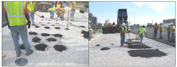
Figure 3-16 - Left: Placing screened asphalt on top of gauges and carefully compacting. Right: Compacting the unscreened asphalt over the gauge arrays with the paving crew approaching.
