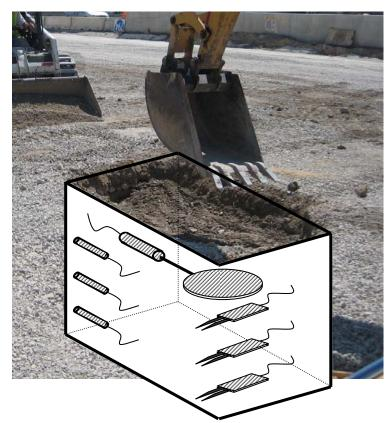
Figure 3-10 - The final arrangement of the sensors after installation. The EPC is aligned so that the sensor leads point into the direction of traffic. All moisture sensors have the pronged end facing east and all temperature sensors have their leads facing north.
