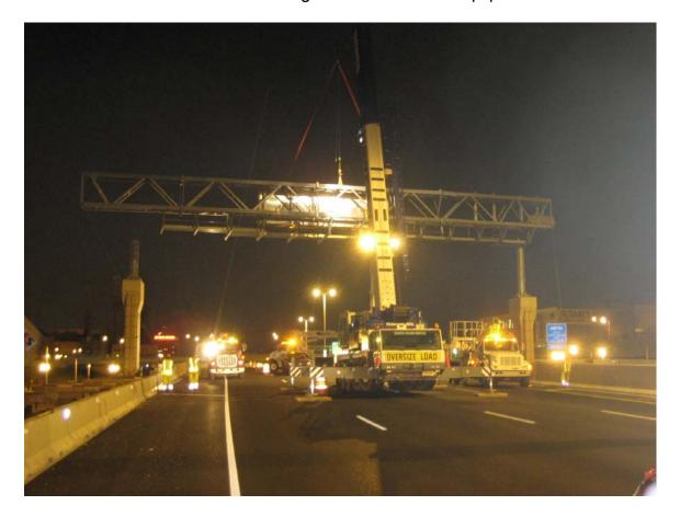
Figure 3-39 - Heavy crane lowering the sign bridge into its final resting position. Note that the outriggers for the crane came close to the sensor locations.
