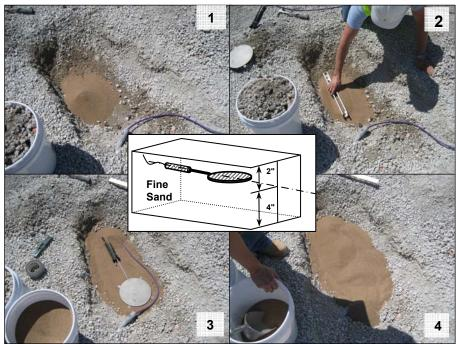
Figure 3-12 - Steps in installing EPC. 1) Filling the cleaned excavation with a bed of fine sand. 2) Leveling the sand out and preparing for EPC placement. 3) Leveling the cell and routing the sensor lead in a safe direction. 4) Backfill against the cell with more sand which would then be followed by the pre-existing base material, compacting each layer by hand. The inset sketch shows the layout of the sensor schematically.
