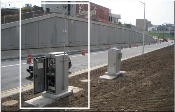
Figure 3-19 - The highlighted cabinet is occupied by the equipment for this project. The mast connected to the cabinet holds environmental sensors as well as the wireless communications antenna. The cabinet in the background houses various traffic control devices for WisDOT. The two cabinets are connected by a limited number of conduits.
