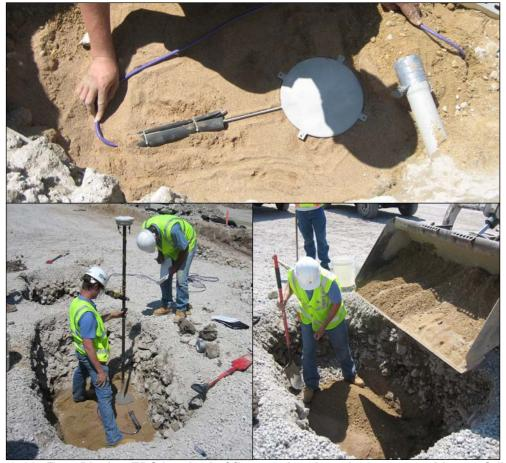
Figure 3-11 –Top: Placing EPC in a bed of fine sand and routing sensor cable carefully. Bottom left: Measuring and recording the final location of the EPC with a GPS based measuring device. Bottom right: Backfilling against the EPC with sand.
