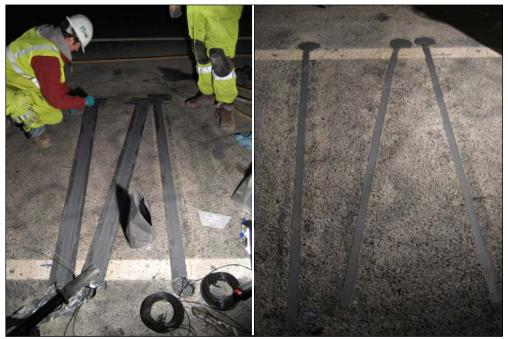
Figure 3-24 - Left: All three wheel-wander sensors have been installed and the grout on the final sensor is being leveled with the pavement surface before hardening. Right: All three sensors installed with the tape removed. Note the pictures have been taken from opposite sides.
