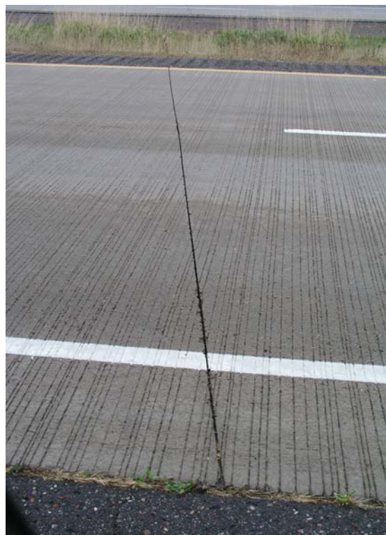
Figure 4.4.5 Typical Chipped Joint – WIS 29 Abbotsford
