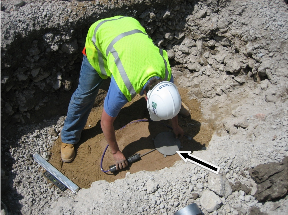
Figure 4-12 - Earth pressure cell installation.
