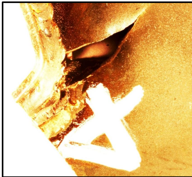
Figure A7. Photo of the crack sectioned at the end of test of Specimen 4.
