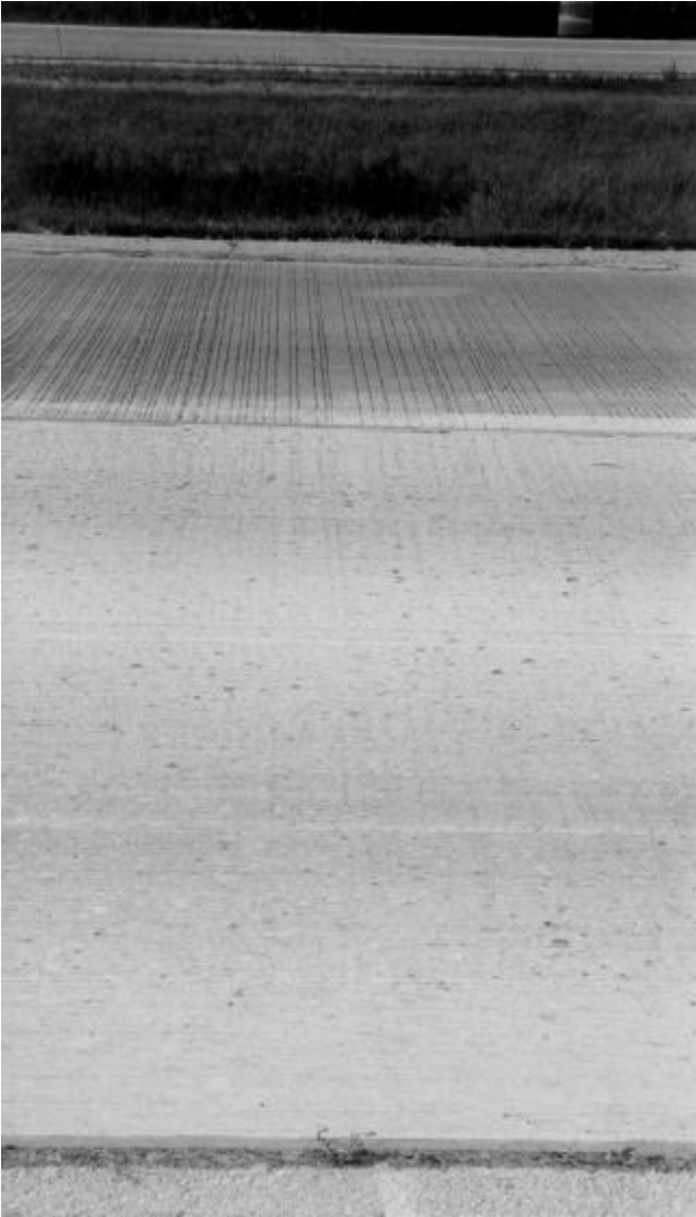
Figure 1a – Inside lane transversely tined. Outside lane diamond ground.
