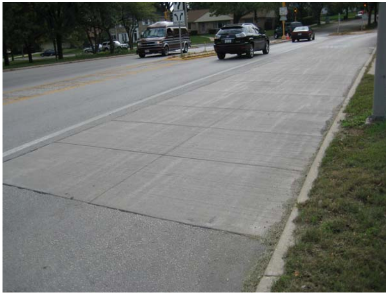
Figure 3.1: 87 th Street Bus Pad Test Section, Looking North
