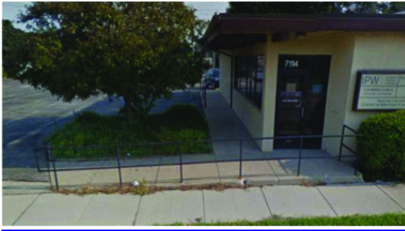
Fig. 9. Wrong classification of the building with a ramp.
