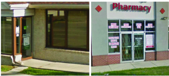
Fig. 8. Wrong classification of buildings' accessibility.
