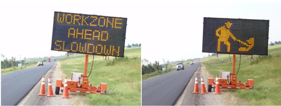
Figure 1. Text-graphic PCMS with the Work Zone Graphic (from Huang and Bai (2014) Figure 3, license obtained)
