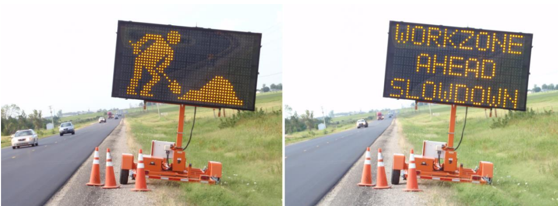
Figure 6. Text-graphic PCMS with Work Zone Graphic Alternative One (from Huang and Bai (2014) Figure 9, license obtained)
