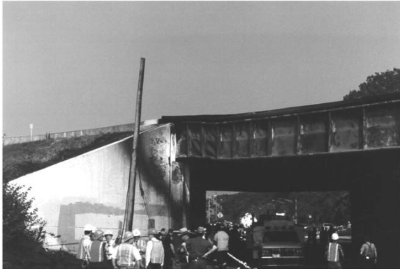
Figure 1: Overview of the damaged I-87 Bridge
