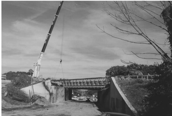
Figure 2: Two prefabricated steel truss bridges for temporary traffic detour
