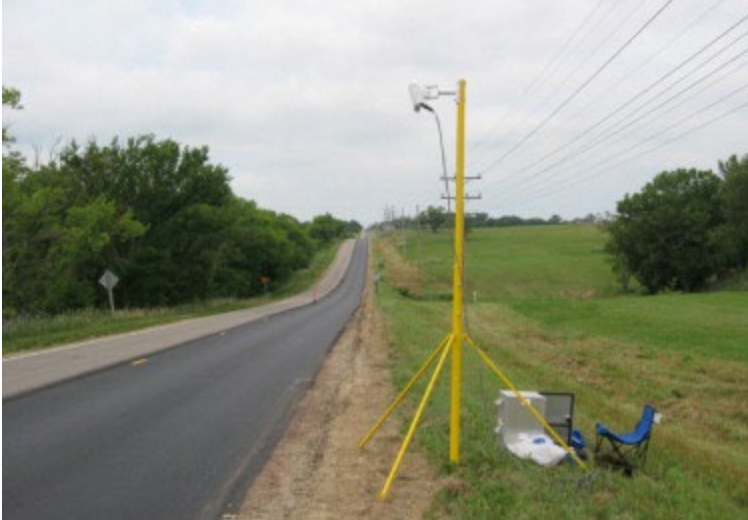
Fig. 1. A speed detector sensor installed at an experimental site.
