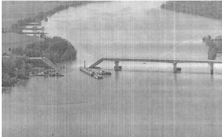
Figure 2. Overview of damaged bridge
