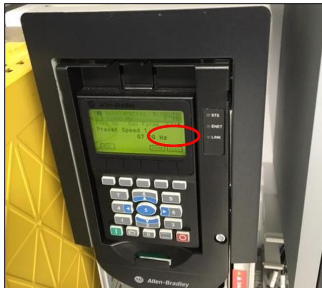
Figure 68: PowerFlex Drive showing the parameter changes to increase the speed
