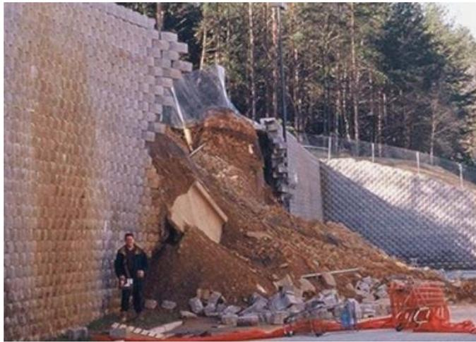
Figure 1.4: MSE wall collapse [40]
