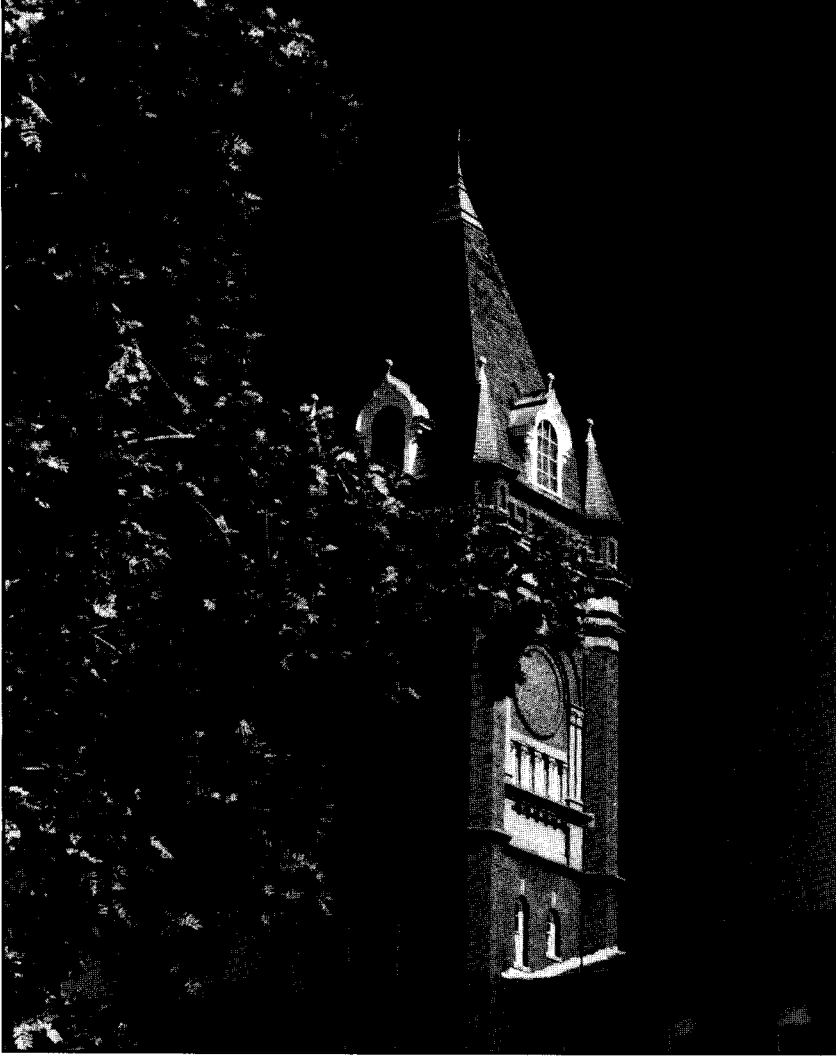
O'Kane Hall, dedicated to the memory of Rev. Michael A. O'Kane SJ, president of Holy Cross from 1889 to 1893, was constructed in 1895.
